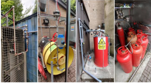
Automatic ammonia-hydrogen ( NH_3/H_2 ) combustion system
